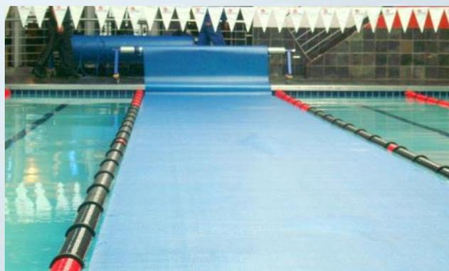
*Single lane thermal cover on gym pool with standard Mercury Rollup Station*
